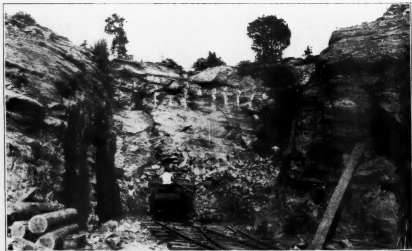
View of New Dallas Quarry—Stone Is Hand Picked and Loaded Into Dump Cars
